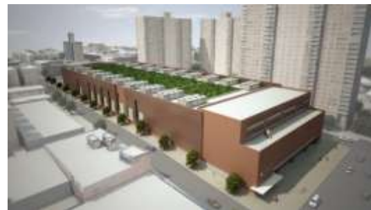
Figure 2: Rendering of the New York City Bus Depot showing its south face and both the corrugated metal and brick veneer facades. (Image courtesy of STV Inc.)
